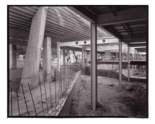
Figure 7. IIT State Street Village, Chicago, IL. Concrete structure of southern unit reaches its final height. emporary wooden posts, visible on all floors, support the concrete floors until they reach their final hardened strength. (2002-11.3-22a).
