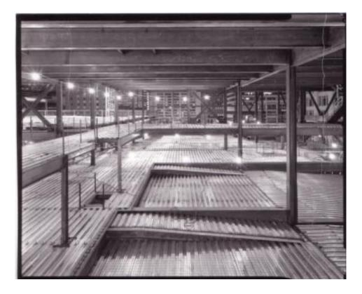
Figure 3. Experience Music Project, Seattle, WA. Structural ribs partially installed in Elements 1 and 2. (1999-5.15-5a).
