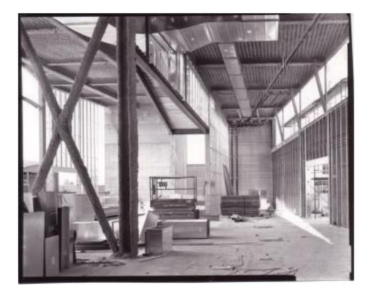
*Figure 5. Milwaukee Art Museum, Milwaukee, WI. Construction of A-frame structure which will later support the building's signature wings. (2000-8.3-9a).*
